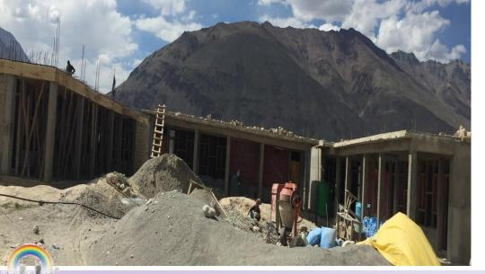
We have completed the outer plaster for two building and about to put the roof on third Building, after that we will level the surface around the main building and remaining plaster inside out and all the finishing like paint, wooden flooring, and classroom decoration etc.
