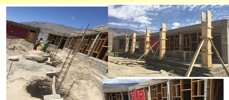
we started with varendha and lintel pillar, as the weather was worm and fine, the varendah will provide good pavement for the Students and shade which will protect the windows from direct sun light.
