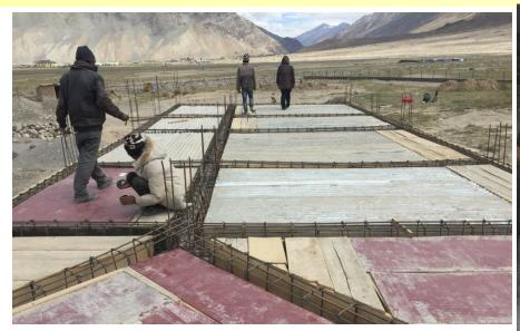
Workmen laying steel reinforcement for concrete slab, as we received more and more rainfall year by year we decided to put concrete slab for the last and 3rd block of the building to avoid any leakage in the room.
