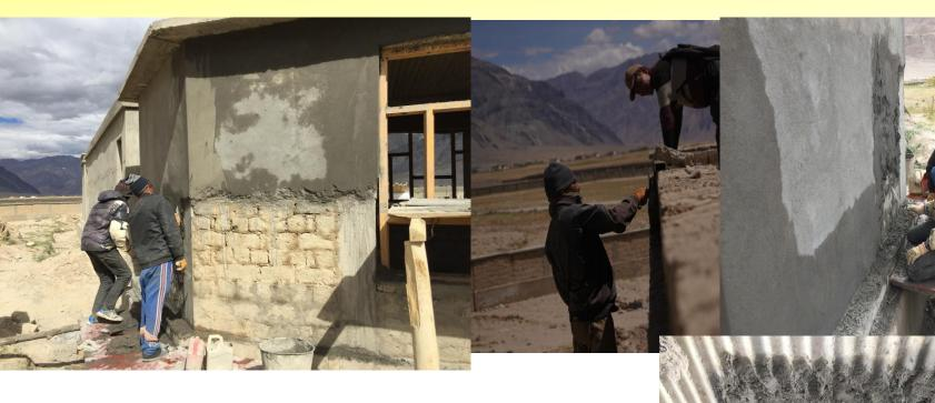
The outer facade of the building are plastered in Cement to resist against rain and Snow and the inner surfare of the Room are plastered with the mixture of Mude, clay, straw, Cowdungs, cement, which is done in taking care of cold climate in the winter, still one layer of plaster inside of the room are yet to finish.
