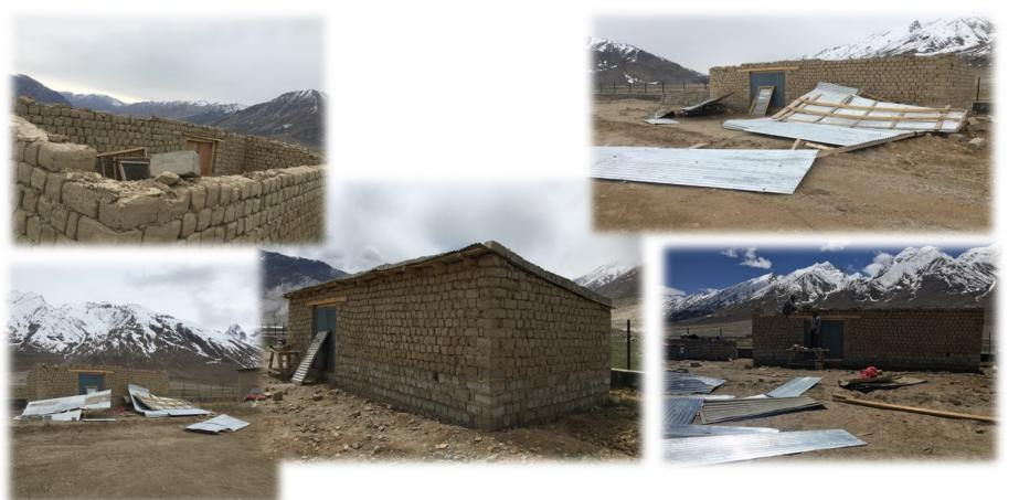
On 10th may a tornado hit temporary store shed and took off the roof which was reinforced with wooden beam and cement bricks on the top. And the very next day we reinstalled the roof as to prepared for Summer rain and
